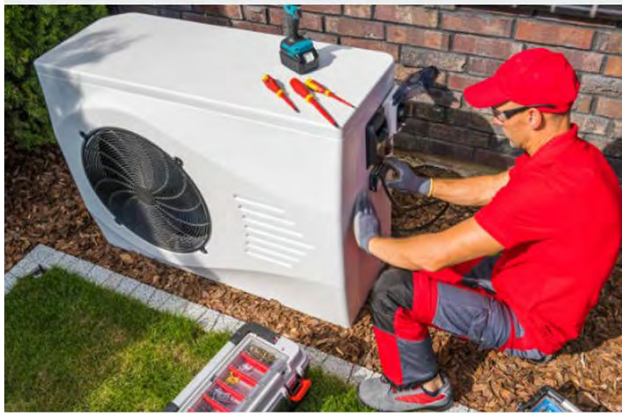
Top: Fuel Assistance Team Front row (Left to Right): Srey Lunn, Sarah Oyola Back row (Left to Right): Donna Kelly Kamara, Vanessa Plante, Chenda Rous, Mary McKenney Bottom: Energy and Weatherization staff member installing a new Air Source Heat Pump (ASHP).
